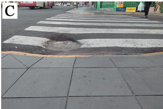
Figure 2 - Holes in the safety lane in the image on the left and in the sidewalk in the image on the right.
