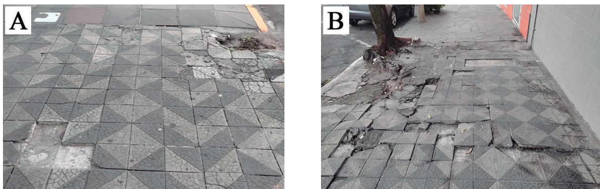
Figure 1 - Lack of paving stones, hydraulic tiles, on the sidewalks in the area.
