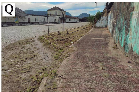
Figure 9 - Lack of lowering of sidewalks in the square and in front of the Railway Station.
