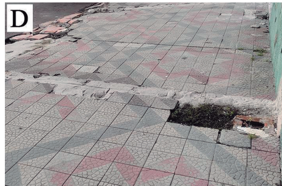
Figure 2 - Holes in the safety lane in the image on the left and in the sidewalk in the image on the right.
