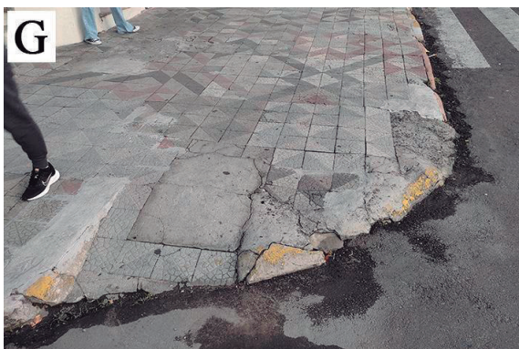
Figure 4 - Access ramps not in line with technical standard guidelines.
