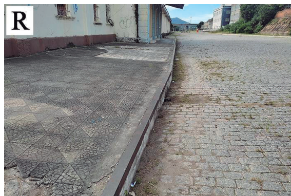
Figure 9 - Lack of lowering of sidewalks in the square and in front of the Railway Station.
